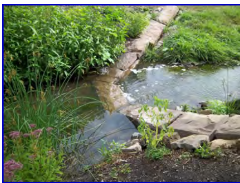
One of two rock cross veins directs flow to the center of the stream to protect the bridge structures.
