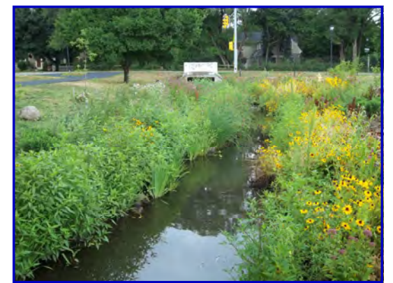
West Segment—July 2012 The riparian vegetation has become well established despite serious drought conditions. The stream meander that was created is also visible.
